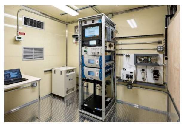
The client said Cemtek KVB-Enertec's prior excellent performance when supplying CEMS to them was the reason they came back to Cemtek for CEMS on the new upgrade. Cemtek will engineer, built, tested, install and certify these CEMS to meet a tight schedule that requires extensive project management. The CEMS will measure NOx, CO, NH3 & O2 and will be meet all local State & EPA rules & regulations.
