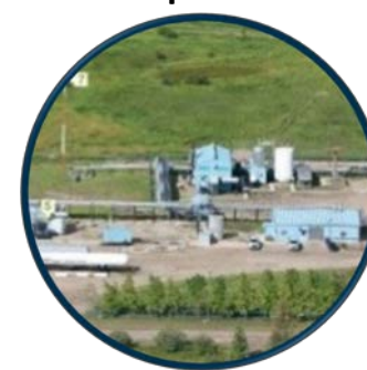
Gas Processing Components
