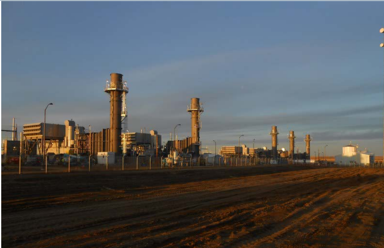
5 x LM6000 SCR systems in operation
